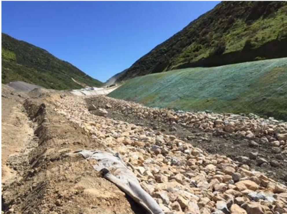
**Horokiri Stream permanent diversion channel under construction (view looking north towards Wainui Saddle)**
