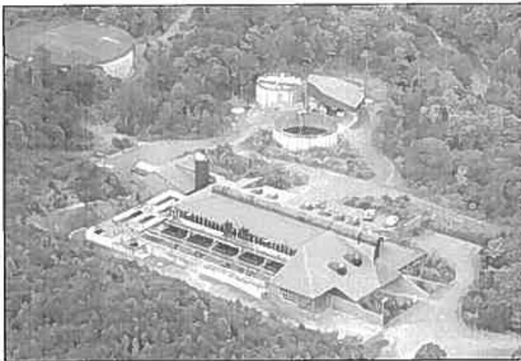
The plant's design capacity is 60 million litres per day but production is typically around 30 million litres daily, or just under 20% of the total supply each year. The Wainuiomata plant supplies water for Wainuiomata and together with the Waterloo Water Treatment Plant, Wellington's business district, and the city's southern and eastern suburbs.
