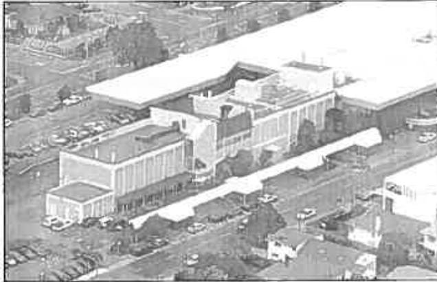
Like Gear Island, improvements are limited to the main building which incorporates all facets of the water treatment process, together with supporting control room, staff facilities, motor room, electrical and workshop facilities. More recently, an enclosed lean-to garage type structure containing the mobile emergency generator has been constructed to the rear.
