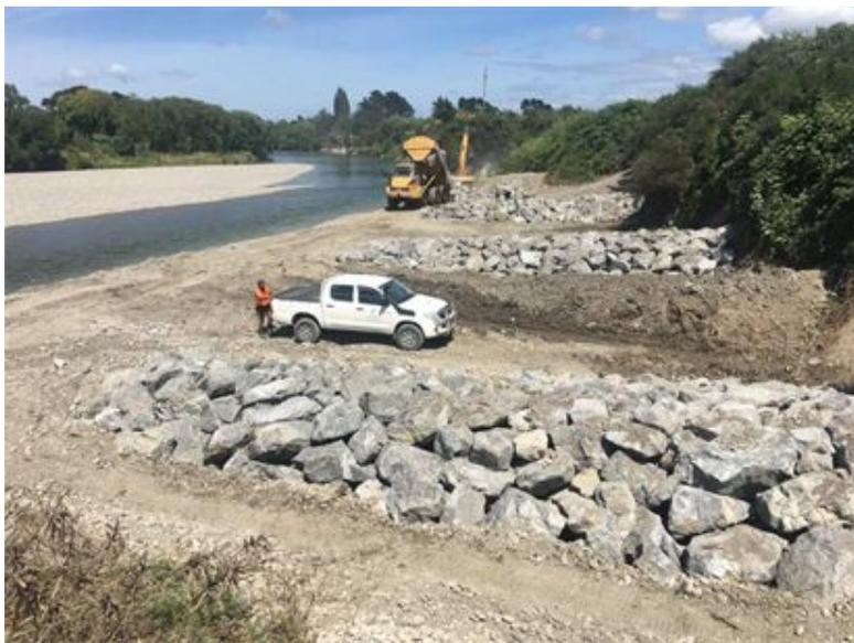
*Photo 5: Dakins Road completed rock groyne construction.*
