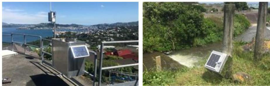
**Left: Rain gauge installation at Ngaio Reservoir. Right: Hydrological monitoring site at Owhiro Stream.**
