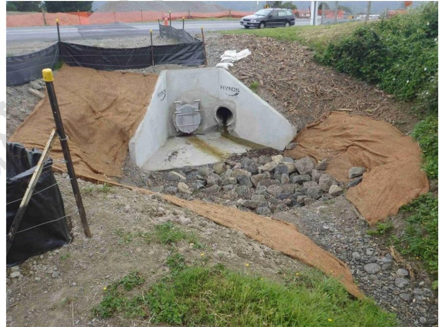
*Silt fencing and ground stabilisation around newly installed wingwall*
