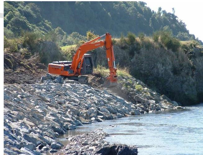
*Placement of rock; machine working from the bank*
