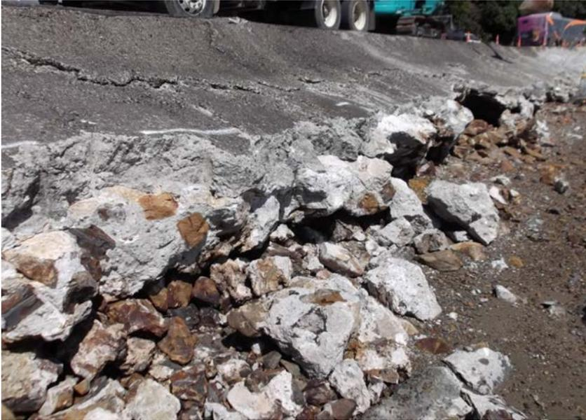
Figure 4-1: Removal of sections of existing seawall
