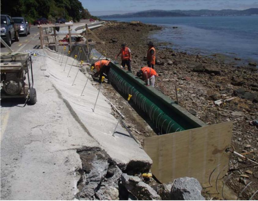
Figure 4-3: In situ concrete pouring using shape formers (lower section)
