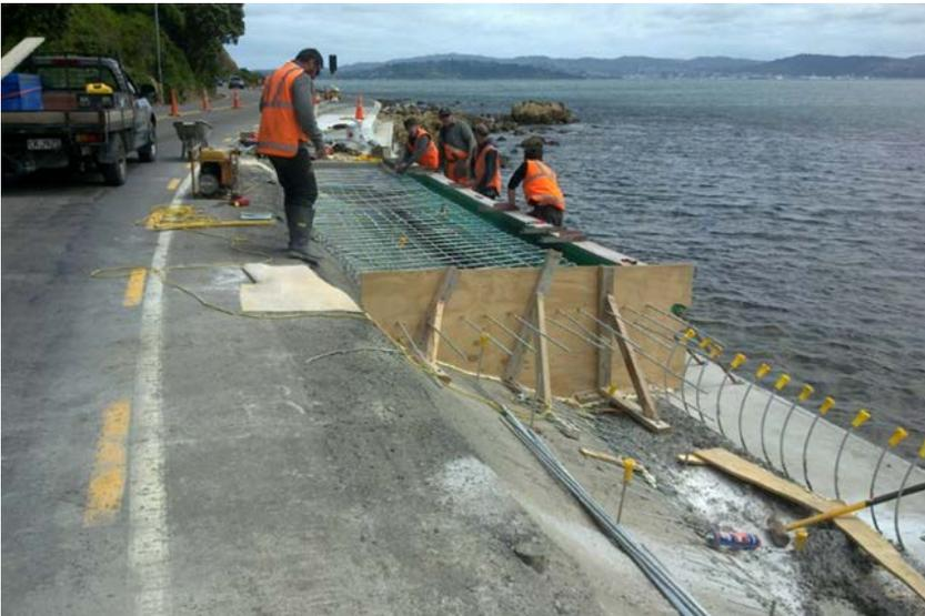
Figure 4-4: In situ concrete pouring using shape formers (upper section)
