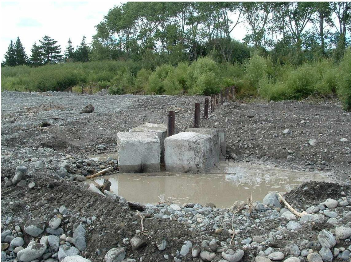
**Figure 5-4: Completed debris fence (Otaki River)**
