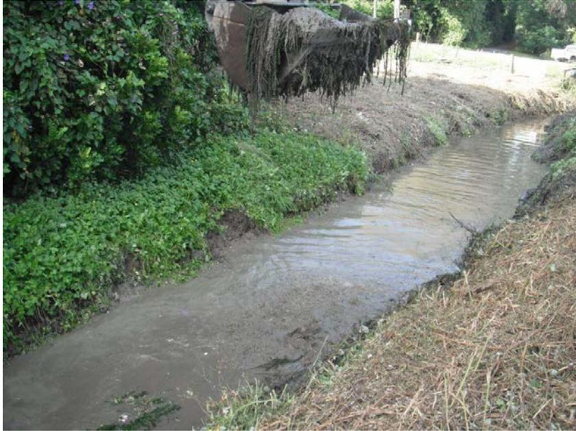
**Figure 5-6:** Vegetation clearing in Waimeha Stream by digger fitted with a 'weed bucket'
