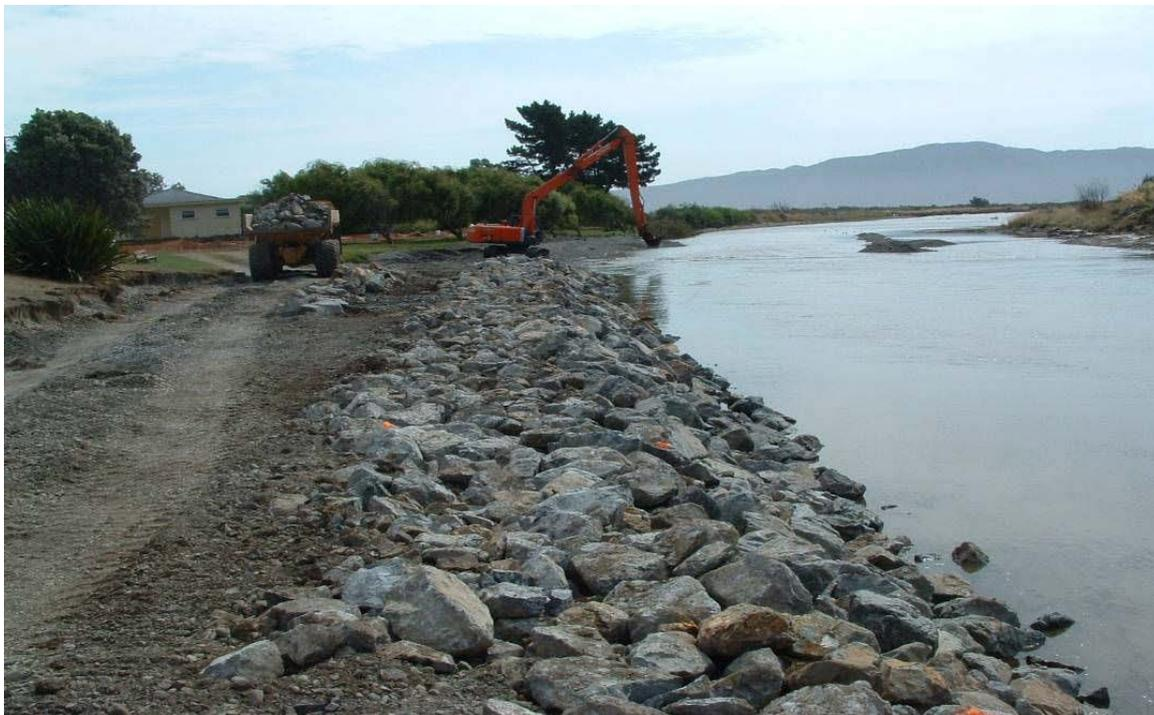
**Figure 5-3: Rock rip rap construction on the Waikanae River at Otaihanga**
