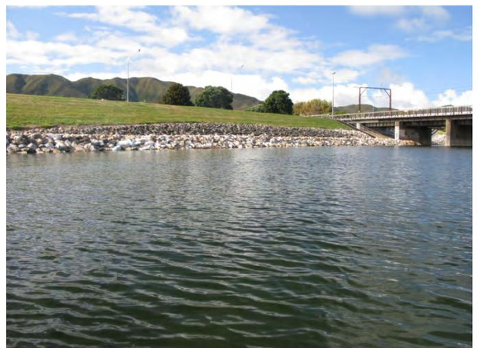
**Figure 17.** Looking downstream at a section of the Hutt River that is protected by anti-scour
