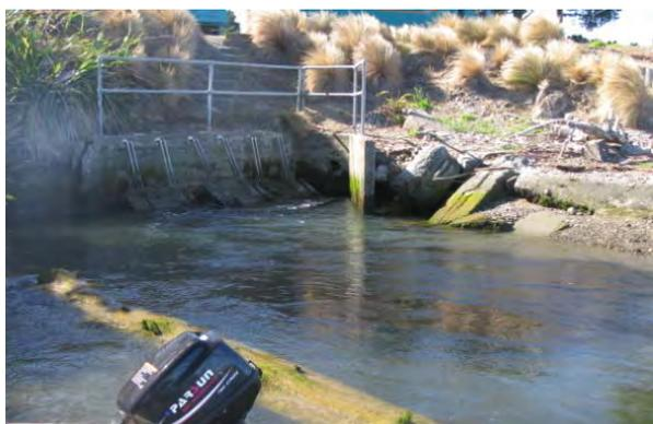
**Figure 19b.** Looking upstream (from the Hutt River side) at the flap valves on Te Mome Stream.
