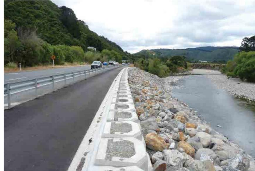
*Erosion protection works adjacent to SH2 to protect the road from being undermined by the river were carried out by NZ Transport Agency in 2017. This section of the Hutt River Trail was reinstated as part of these works.*
