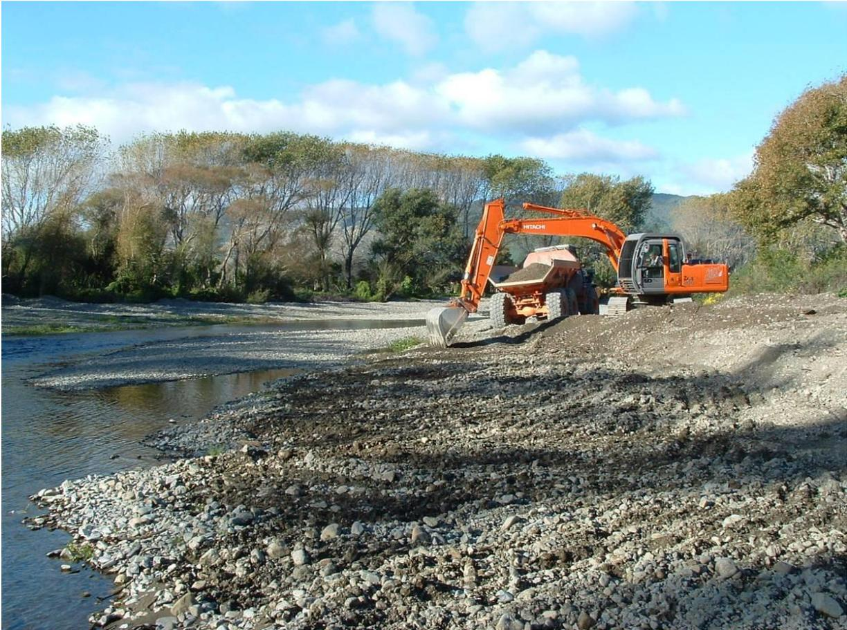
Figure 11: 'Dry' extraction from beach above active channel (Waikanae River)
