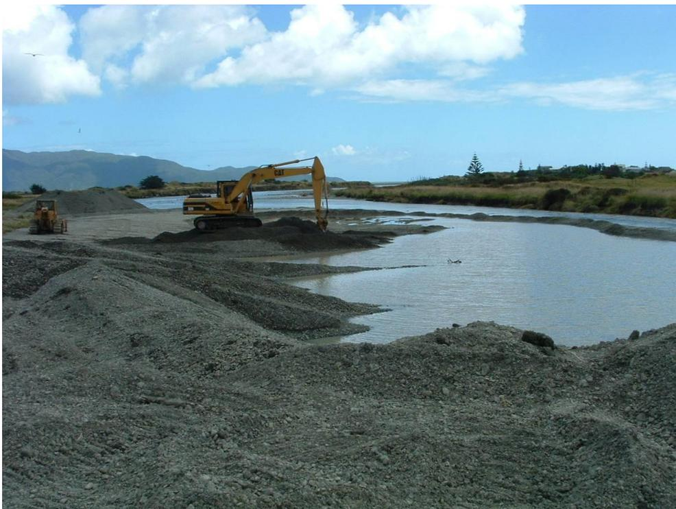
*Figure 13: Extraction of gravel from the tidal reach (XS 60 approximately)
