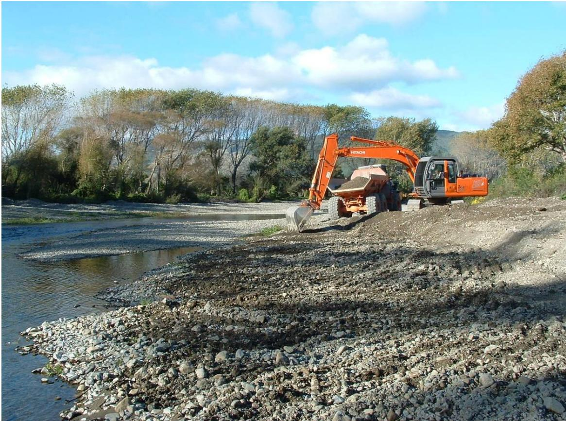
Figure 14: 'Dry' extraction from beach above active channel
