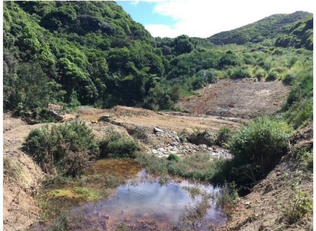
**Figure 3-4:** Wetland treatment system under construction at toe of landfill
