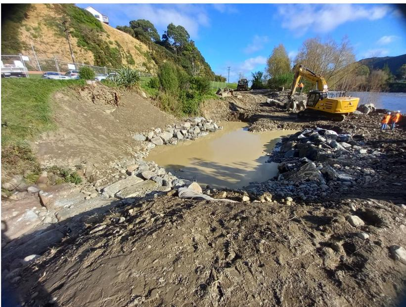
*Figure 2: Site 1 Stokes Valley – Photo of the weir reconstruction*
