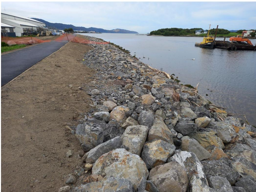
Figure 4: Site 11 Port Road, Seaview – Rock revetment and cycle trail
